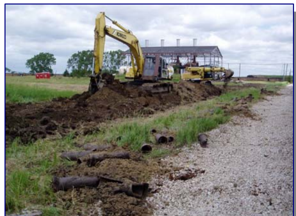
CLAY SEWER PIPES
